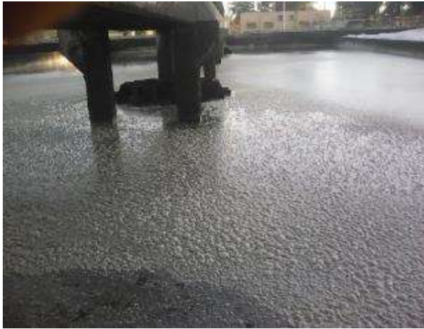
BNR before BioSol SL36 added. The water had a dark colour and foam levels high.
